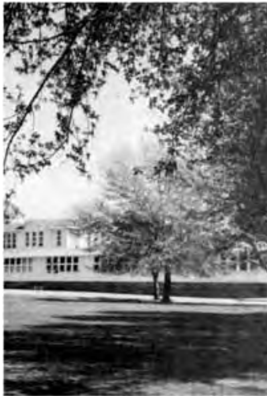
Old Art Block (Demolished to make way for three storey block)
