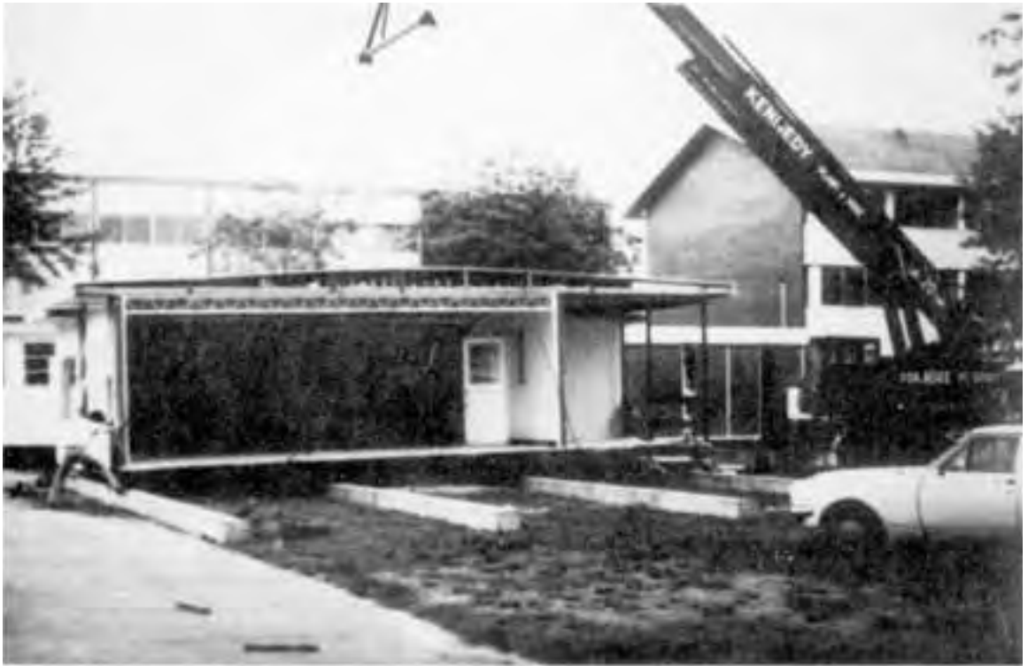
Erection of Temporary Canteen (1975) to make way for the new Library.
